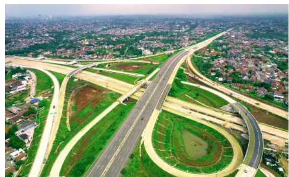
Cinere-Jagorawi 3rd Section Toll Road Project
