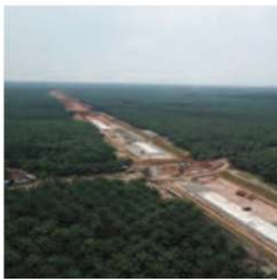
Indrapura Kisaran Toll Road Project
