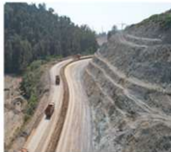
Realignment Hauling Road
