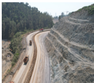
Realignment Hauling Road
