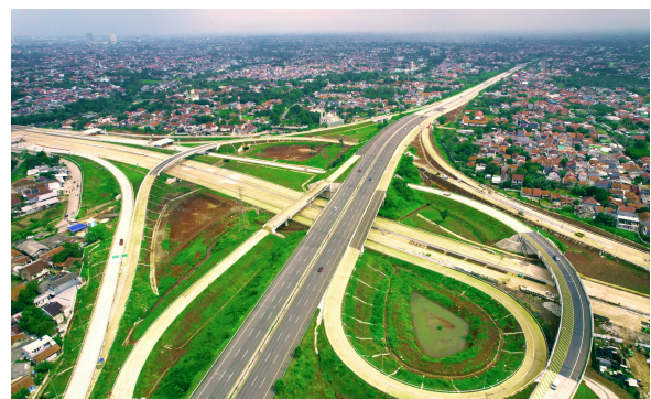
Cinere-Jagorawi 3rd Section Toll Road Project
