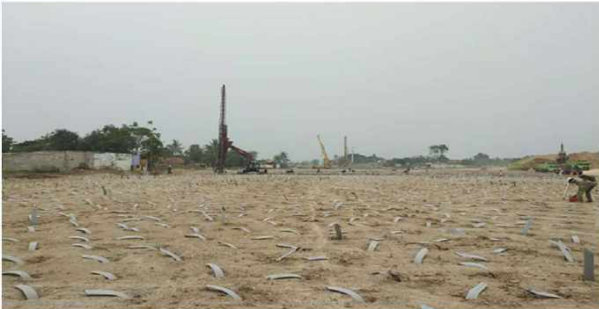
Prefabricated Vertical Drains (PVD) The 3 rd runway Soetta International Airport
