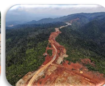
Hauling Road Maintenance Tofu IDR 428.9 M
