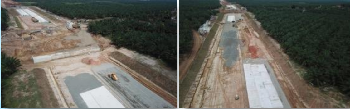
TOL INDRAPURA KISARAN – SUMATERA UTARA Indrapura Kisaran Toll Road – North Sumatera
